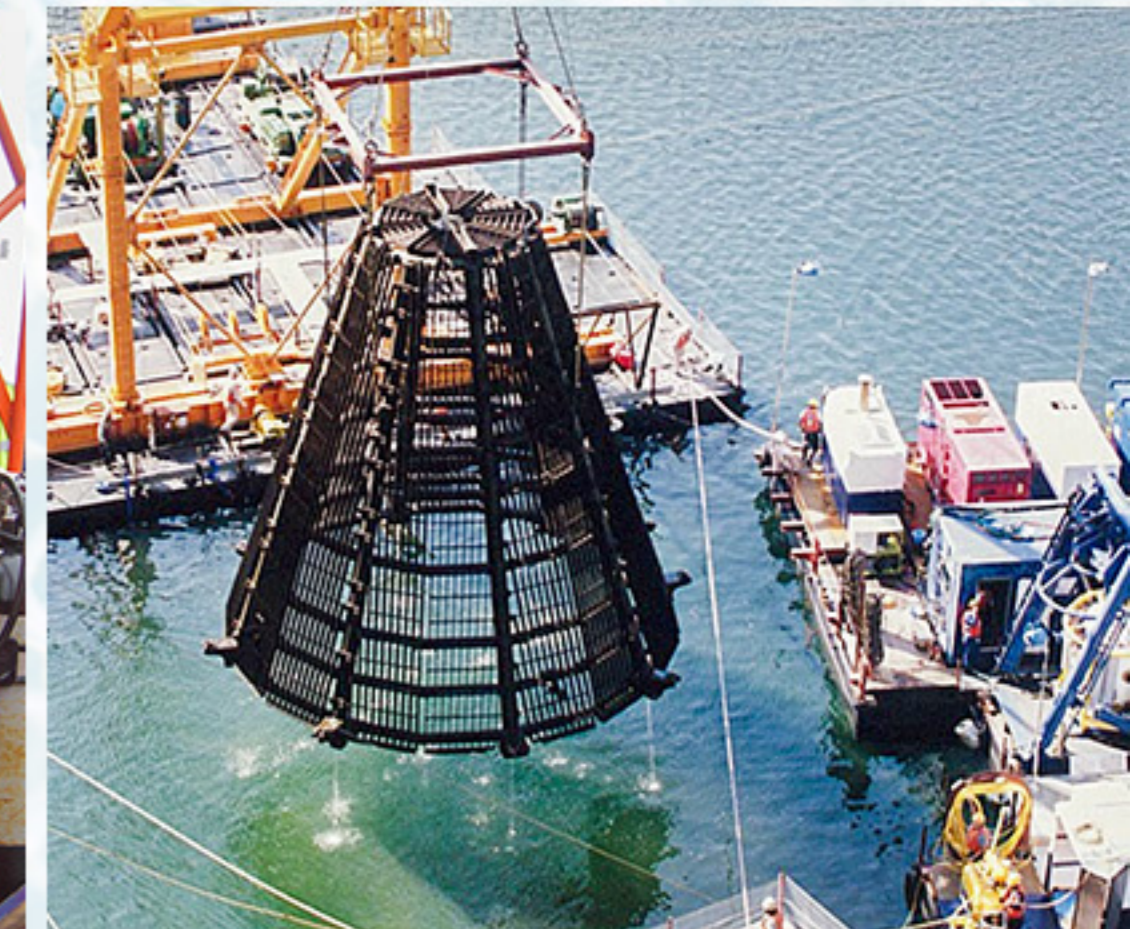
飽和潜水工法によるダム取水塔閉塞工事 Water intake tower installation utilized saturation dam system in a dam reservoir
